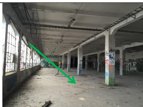
Figur 6. Prov 6. Svart massagolv (asfalt) plan 3 by 18- ej asbest. Låga halter PAH (PAH16 42 mg/kg).
