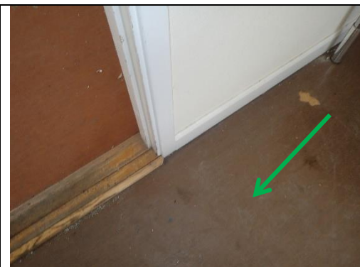
Figur 1. Prov 1. brunrandig PVC-matta by 23-ej asbest.
