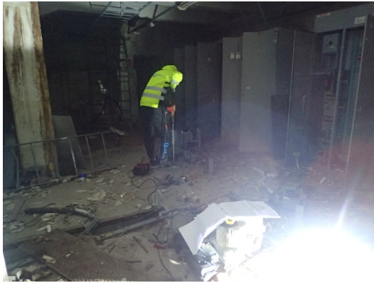
Figur 16. Borrhning genom betongplattor.
